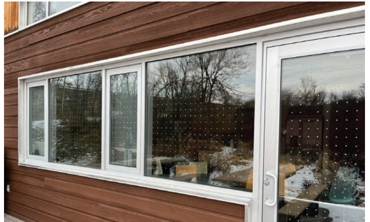
The many windows of the Robert Piper Building are now treated with bird safe CollidEscape dots. The 2" by 2" pattern of dots breaks up the reflection and makes the glass visible to birds. Photos: Paulette Epple
