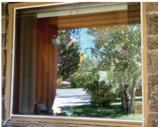
Before and after of a window treated with Feather Friendly Collision Deterrent Marker-Pattern Tape. Taken from the outside looking into the house - note the reflection that so often confuses birds. Photos: Lou Ann Harris
