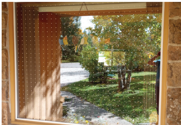
Before and after of a window treated with Feather Friendly Collision Deterrent Marker-Pattern Tape. Taken from the outside looking into the house - note the reflection that so often confuses birds. Photos: Lou Ann Harris
