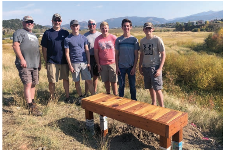
Eagle Scout Troop 0636 poses next to one of three benches they installed along the IAWP Milwaukee Railroad Berm Trail. Photo by Loreene Reid.
