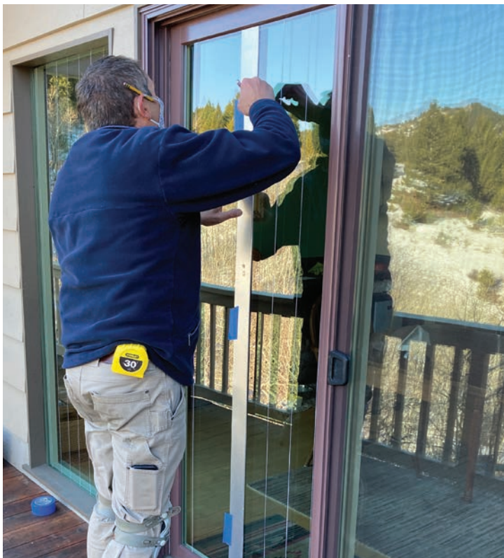
Applying pin stripes with a paint pen and straight edge.
