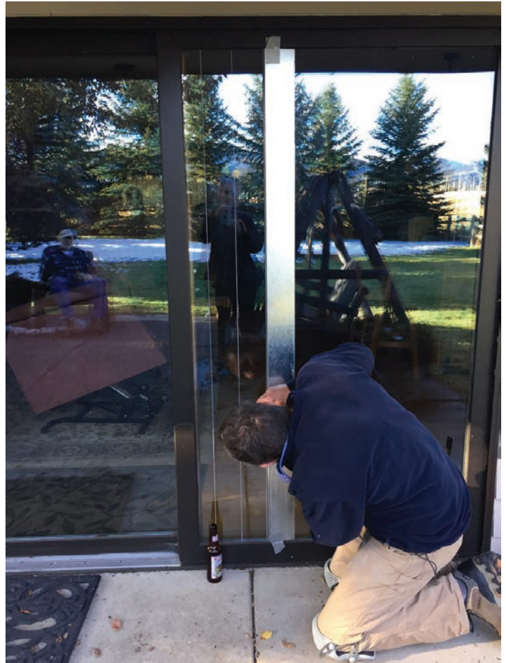
Above: Installation of paint lines with a straight edge. White paint lines are applied 4 inches apart. (Notice the mirror-like reflections!) Below: Acopian Bird Savers or a “Zen Curtain.” Photos by Beth Madden.
