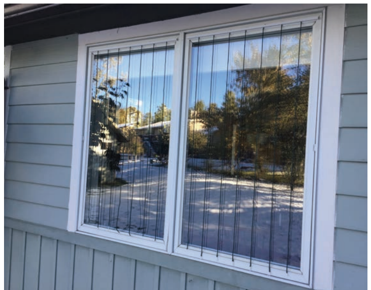
Above: Installation of paint lines with a straight edge. White paint lines are applied 4 inches apart. (Notice the mirror-like reflections!) Below: Acopian Bird Savers or a “Zen Curtain.” Photos by Beth Madden.
